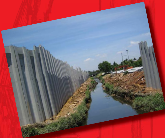
Abutment / Slope Protection
