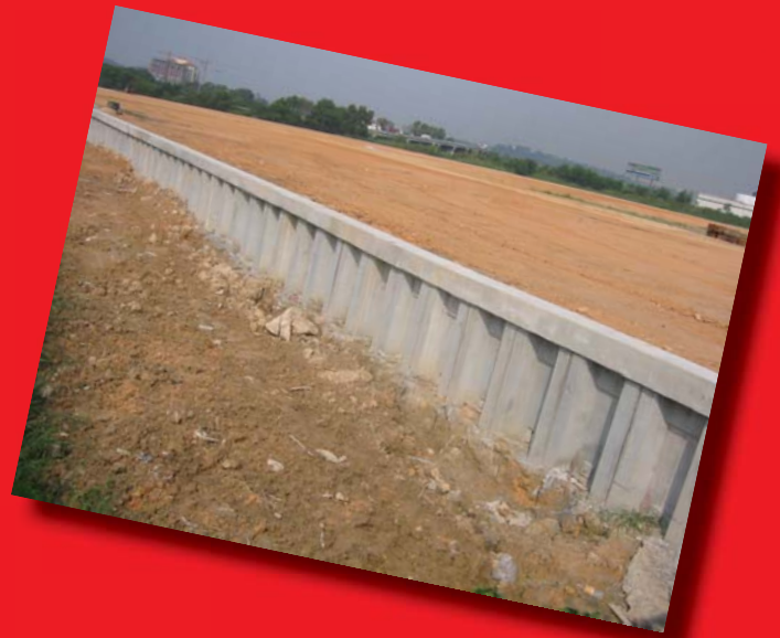
Platform / Earth Retention
